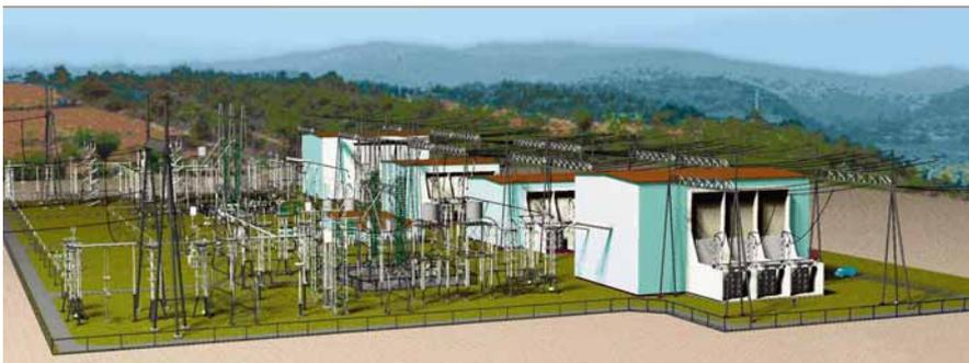
**8** An HVDC converter station with two poles each consisting of two series connected groups
