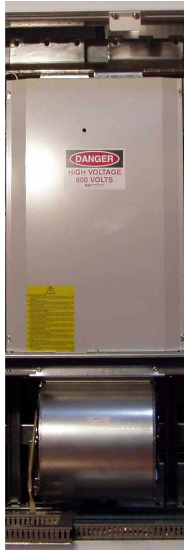
Picture shows ACS600 inverter module used in the fuel cell PCS enclosure.
