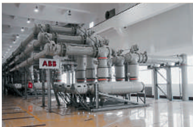
6 Gas Insulated Switchgear (GIS) installed in the powerhouse.
