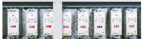
ACH180 is ideal to control fans in air handlers, fan arrays and cooling towers.
