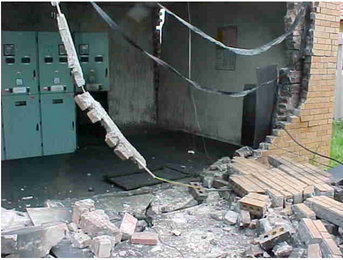
Fig. 3 Arc-fault effect on substation
