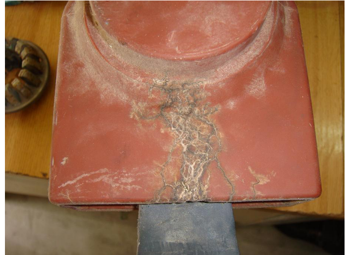
Fig. 1 Overheated insulator with surface tracking
