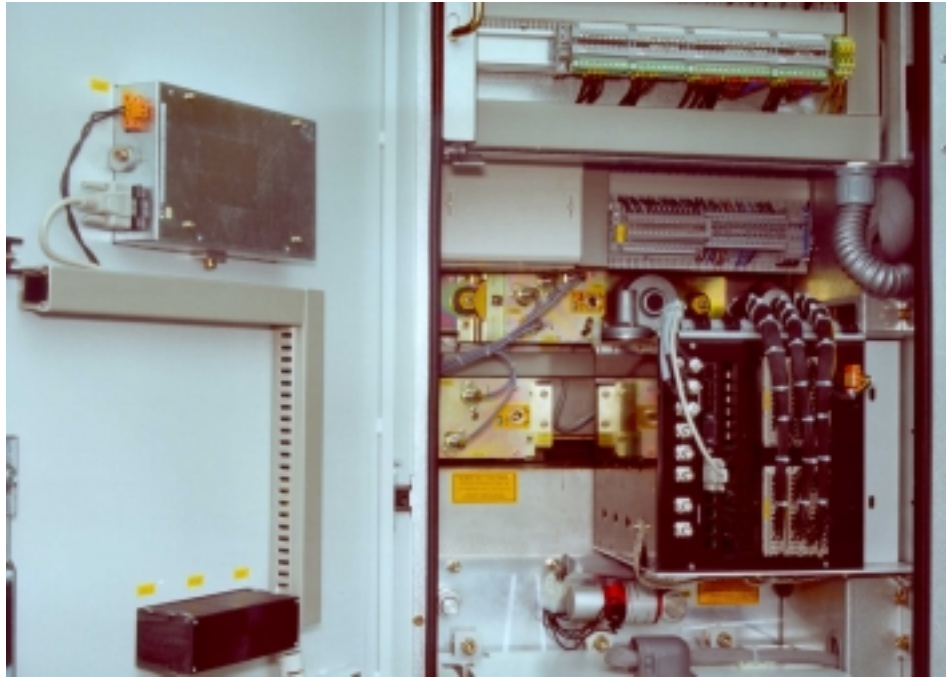
Figure 6: Example of mounting of the Central Unit in the LV compartment and the HMI on the door
