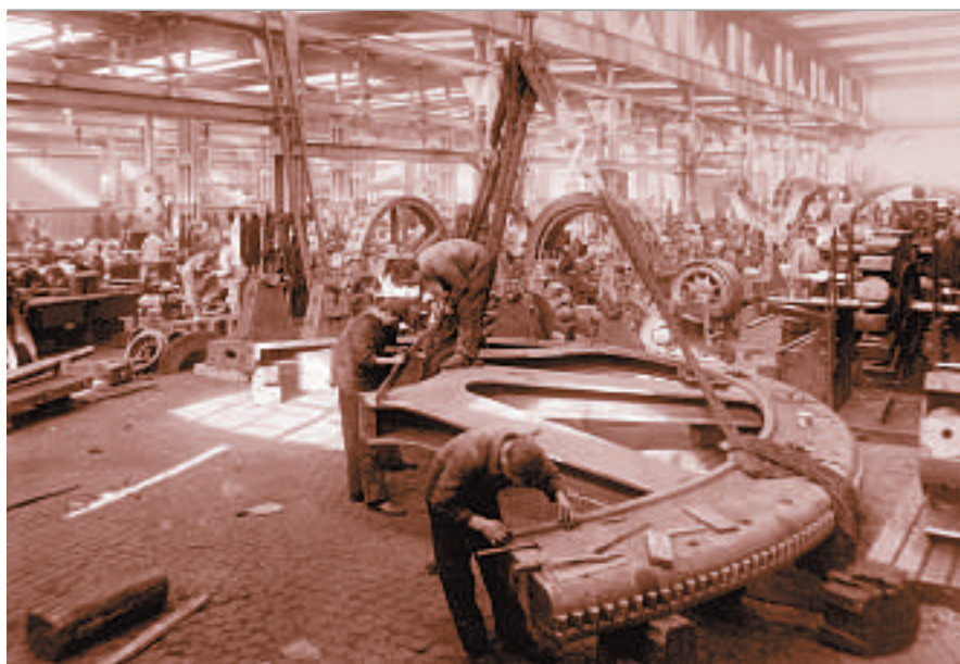
Generator assembly in Baden, Switzerland, 1895
