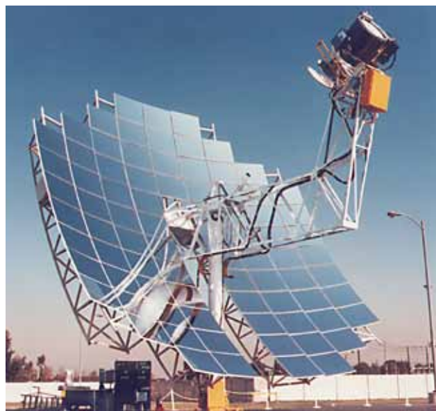
Figure B.6 – Parabolic dish plant
