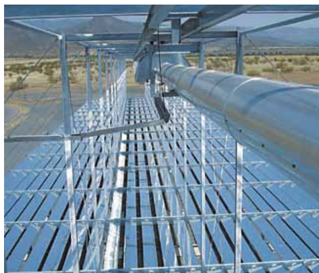
Figure B.7 – Linear Fresnel concentrator plant
