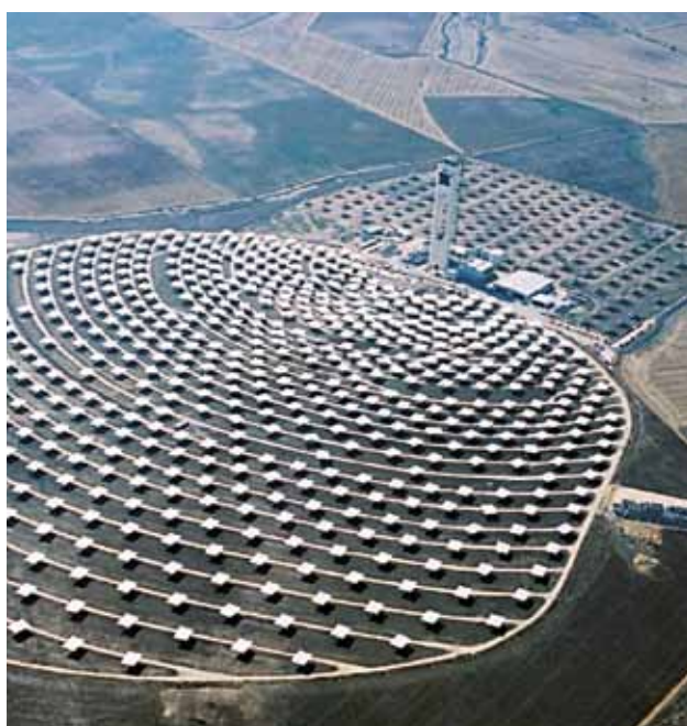
Figure B.8 – Central receiver plant
