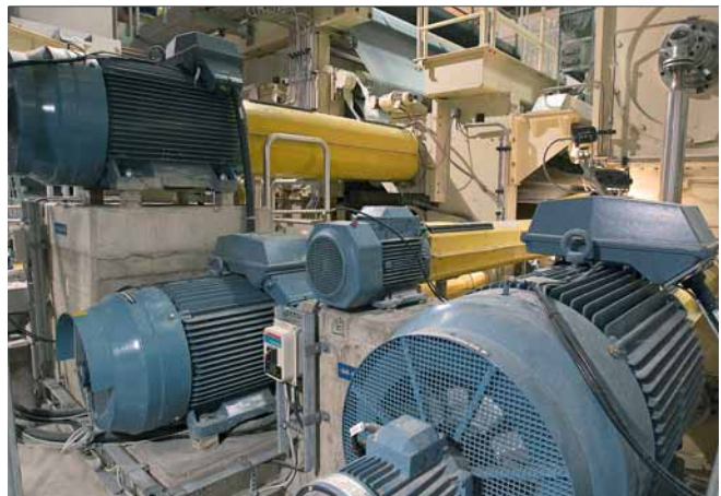
2 The first full-size Direct Drive solution ever installed took place at M-real's Äänekoski mill in Finland
