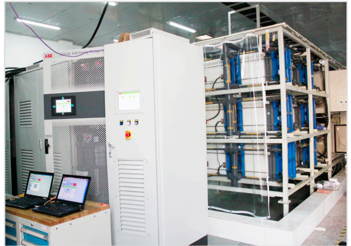
The complete solution of ABB’s PCS100 ESS paired with Prudent’s VRB Energy Storage System
