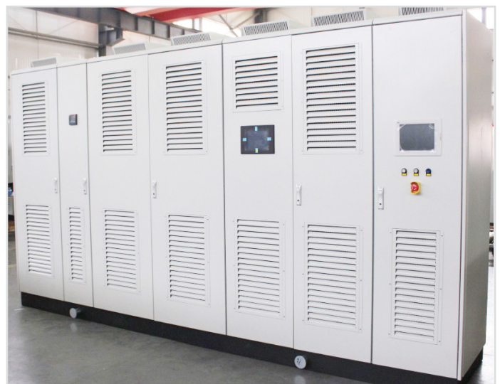
ABB’s 2 MW PCS100 ESS that will help complete the energy storage function with Prudent Energy
