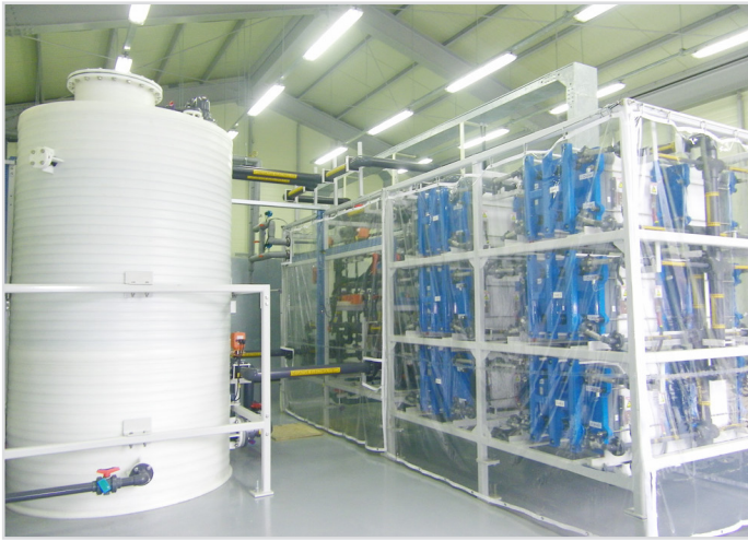
ABB's PCS100 ESS and Prudent's VRB Energy Storage System that has been installed on Jeju Island located in between Korea and Japan
