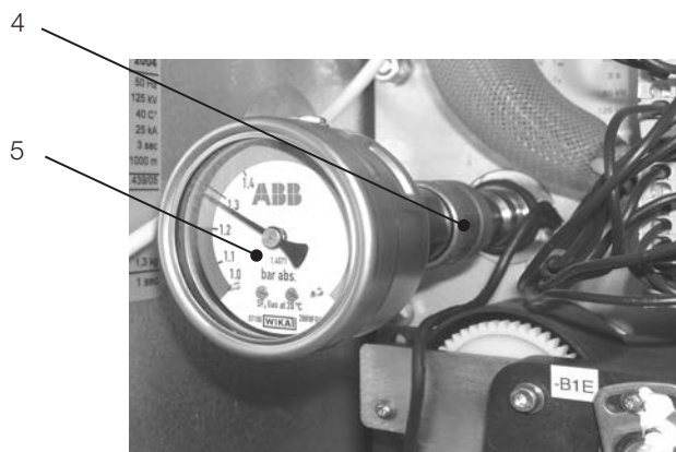
Fig. 2.3.1.1.3: Filling connector with pressure gauge (5) and locking ring (4)
