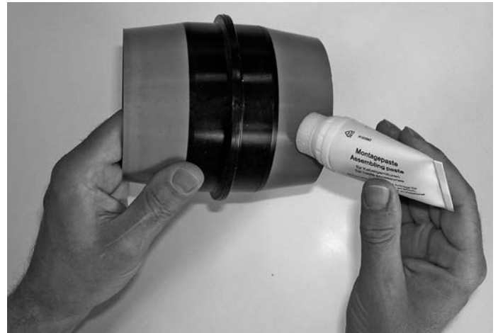
Fig. 2.1.3.1: Greasing the light, outer areas of the silicone insulating part on the busbar connection
