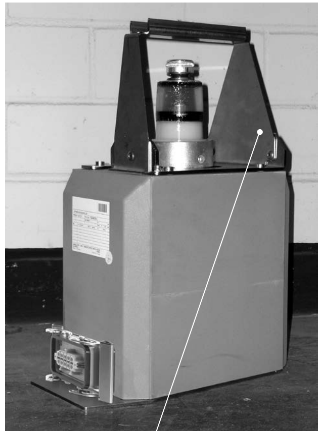
Fig. 2.3.7.1.7: Voltage transformer with lifting handle
