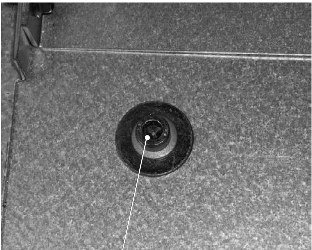
Fastening of the panel to the foundation frame
