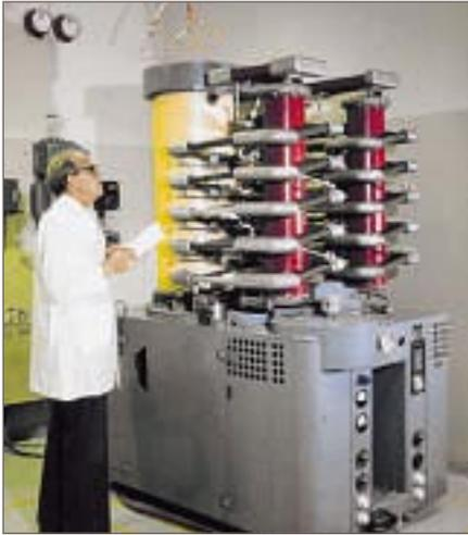
Early mercury-arc valve for HVDC transmission
