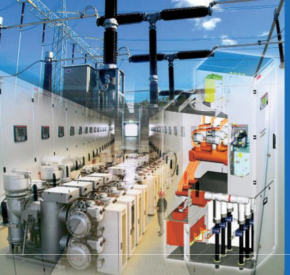
For some time now, SF<sub>6</sub> technology has been used in high voltage switchgears (above 1000 V, as well as in medium voltage switchgears and circuit breakers) in power generation, transmission and distribution plants around the world. The insulating - and extinguishing - gas sulphur hexafluoride  $(SF_6)$  is a nontoxic, non-ozone depleting, non-combustible gas with outstanding electrical properties. However, it belongs to the greenhouse gases covered by the Kyoto Protocol.
