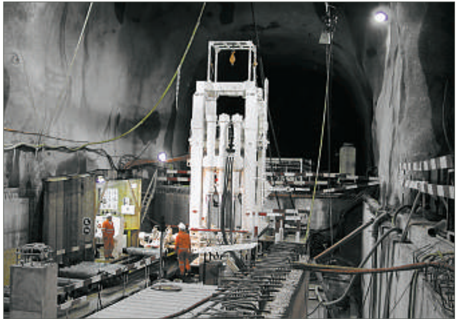
3 Site of the high-pressure pumping station, at the foot of an 800-meters long vertical shaft
