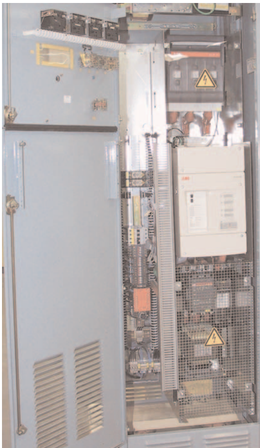
DCE mounted in old cabinet
