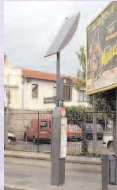
Photovoltaic system at Villeurbanne, France
