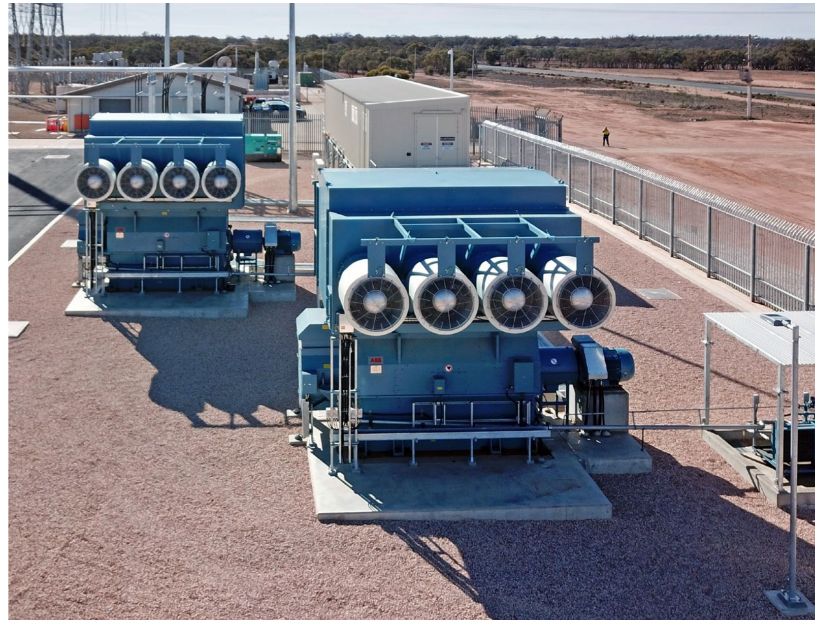
Darlington Point Solar Farm, New South Wales, Australia. This 275 MW solar farm is supported by two air cooled ABB synchronous condensers at its 132 kV connection point (images supplied by Edify Energy and Octopus Investments).
