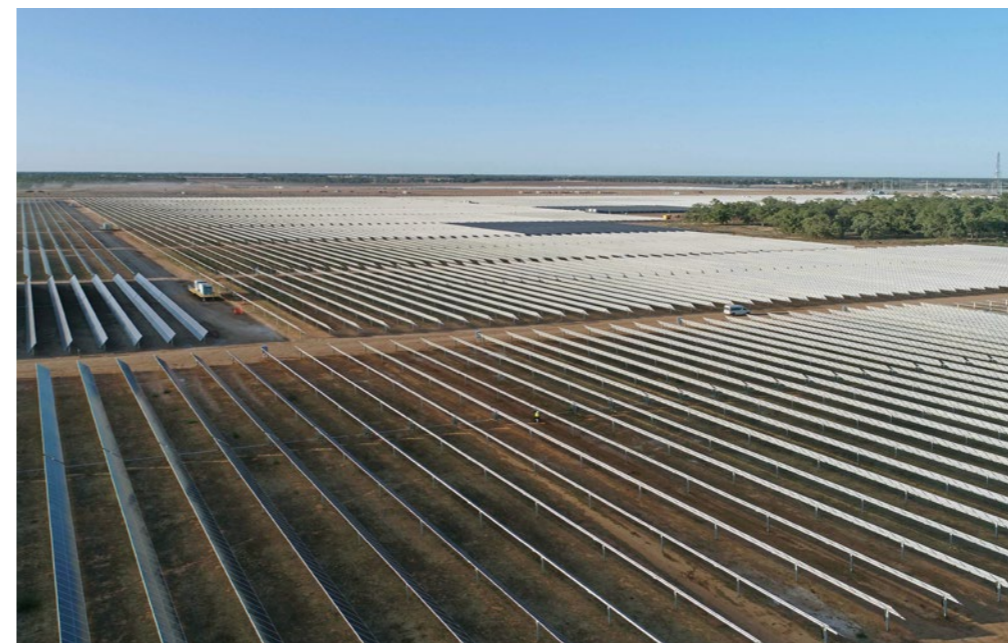
Darlington Point Solar Farm, New South Wales, Australia. This 275 MW solar farm is supported by two air cooled ABB synchronous condensers at its 132 kV connection point (images supplied by Edify Energy and Octopus Investments).
