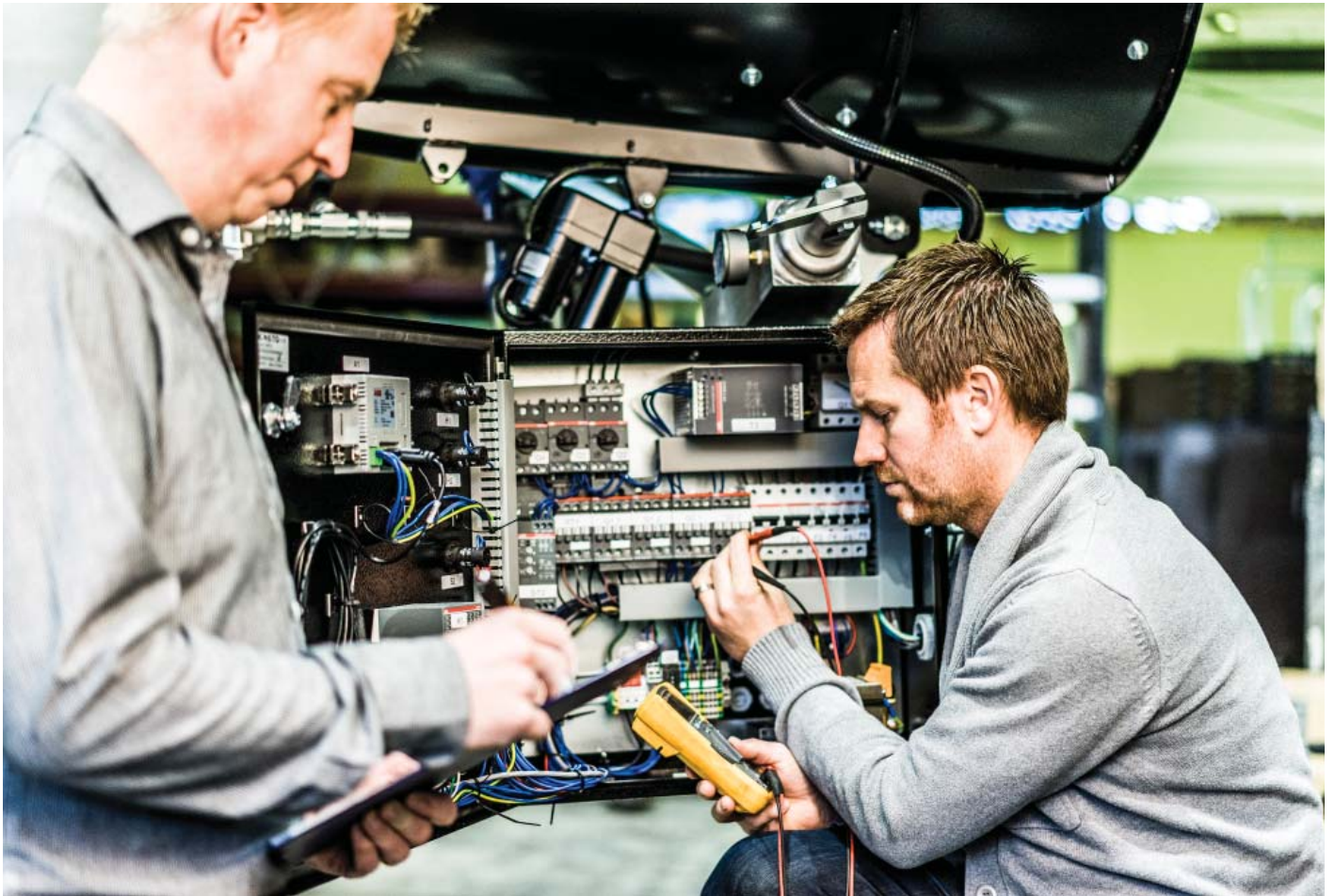
All low voltage products in Duztech's machines are made by ABB, which helps sell quality and reliability
