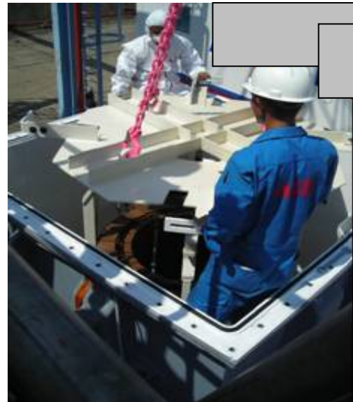
Fig. 13 New windings prepared for shipping in container
