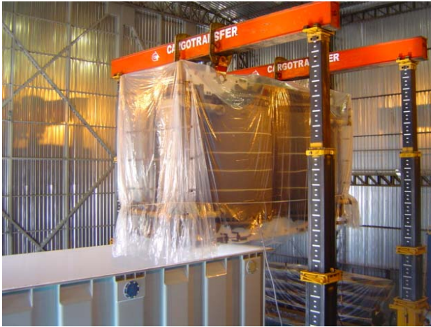
Fig. 6 Tanking of large power transformer using mobile lifting equipment
