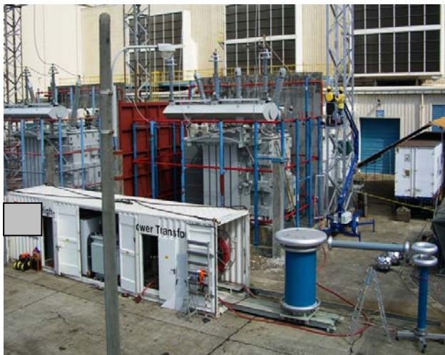
Fig. 15 The Mobile High Voltage Test system set up at site for testing of the repaired transformer
