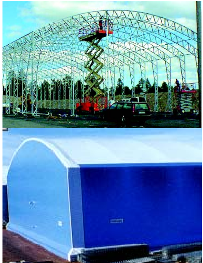
Fig. 5 Typical tent structure that may be used as temporary workshop
