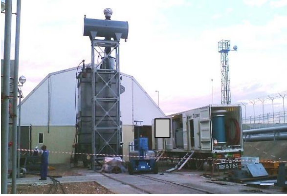
Fig. 11 High voltage testing performed of a power transformer after site repair. The temporary workshop can be seen in the background
