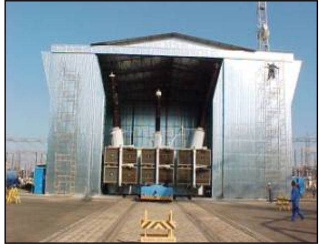
Fig. 4B: A steel building used as temporary workshop in Brazil
