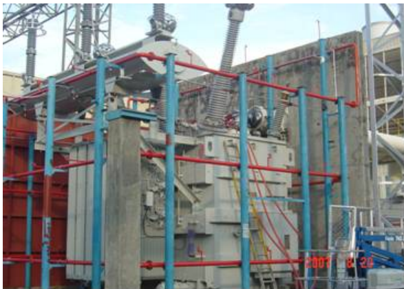
Fig. 12 Transformer on pad, 93 MVA, 240/13.8 kV
