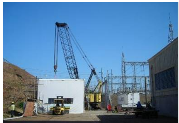
Fig. 14 The temporary workshop set up at site
