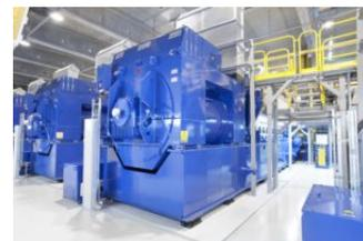
ABB generators on site in Estonia. The plant has a total capacity of 250 MW provided by 25 10-MW generating sets.
