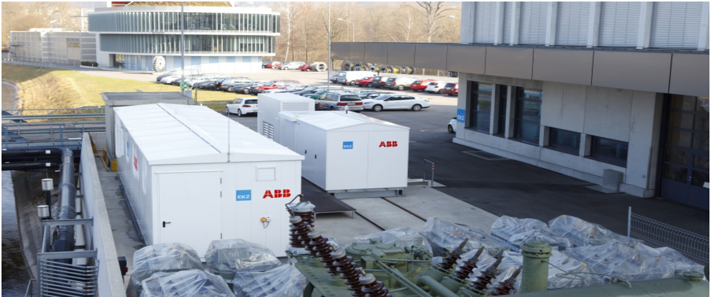
PCS100 ESS 1 MW / 500 kWh battery solution at the Dietikon Powerplant based in Switzerland
