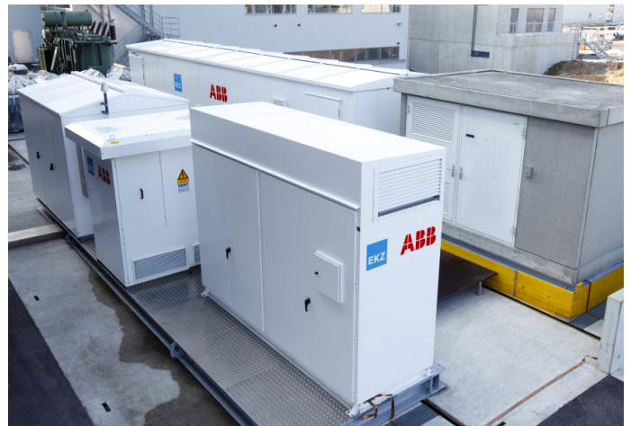
The complete package: PCS100 ESS converter, LG battery, switchgear and transformer
