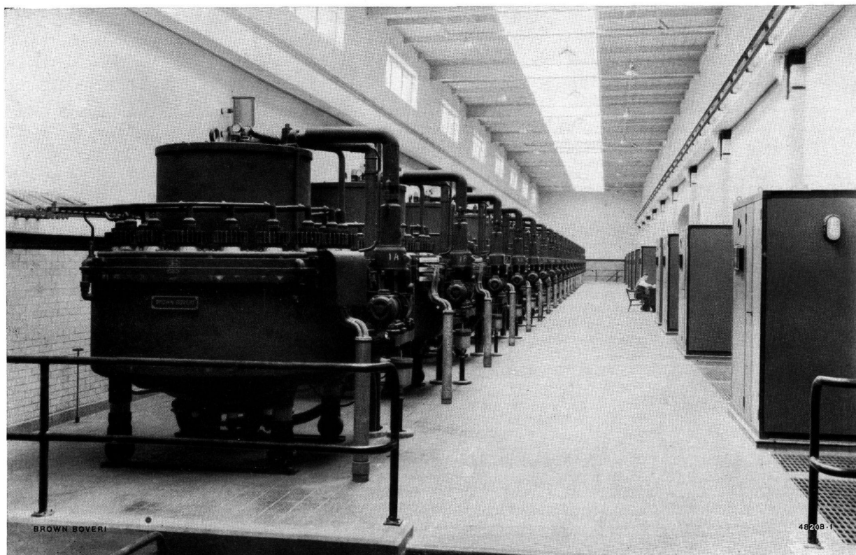
Mutator plant Arvida of the Aluminium Company of Canada.
