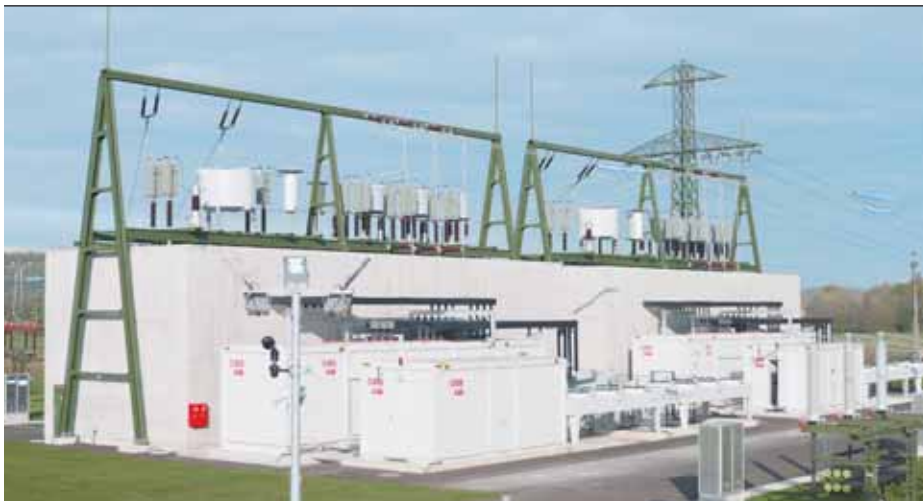
The two × 30 MW converter station in Timelkam, Austria
