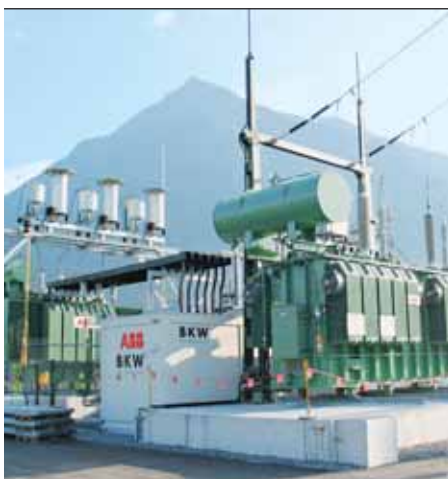
3 The Wimmis converter station for the new Lötschberg rail tunnel
