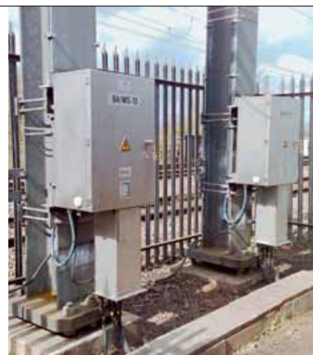
1b New electronic controller at ground level
