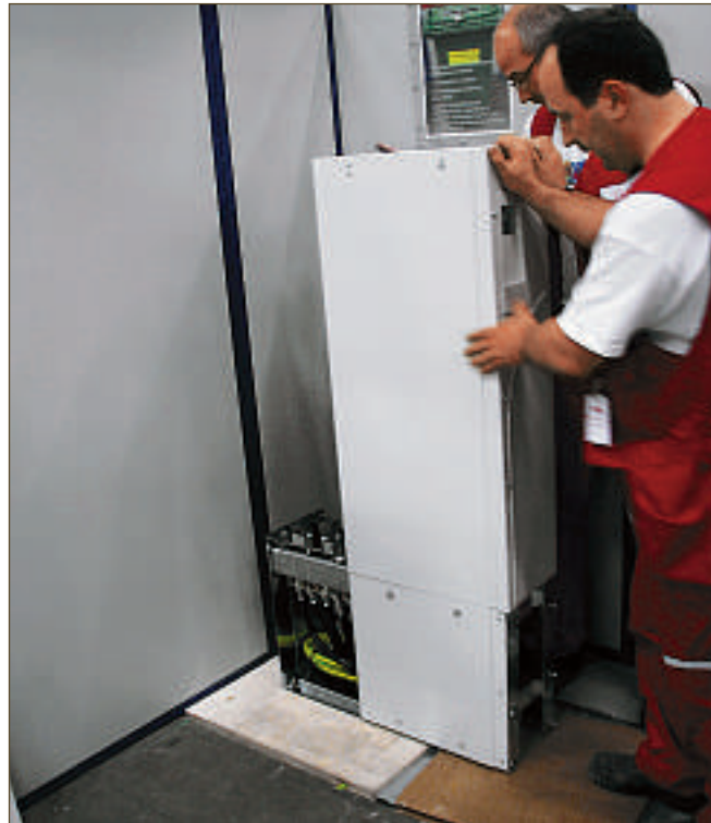
3 After the cabling has been completed, the drive is wheeled over the pedestal and then locked into position.
