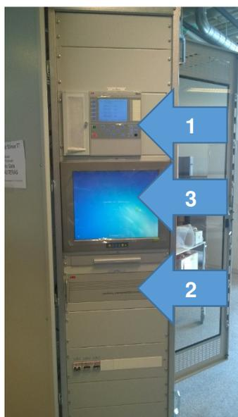
Figure 8: New SSR protection panel for Forsmark NPP
