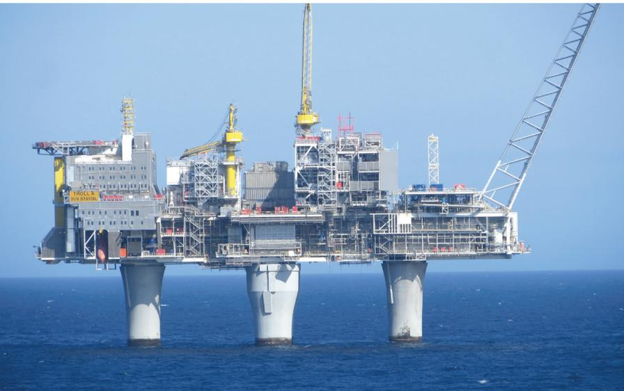
Troll A is a majestic construction, 472 meters high, with an underwater concrete structure to 369 meters depth and a dry weight of 656 000 tons.
