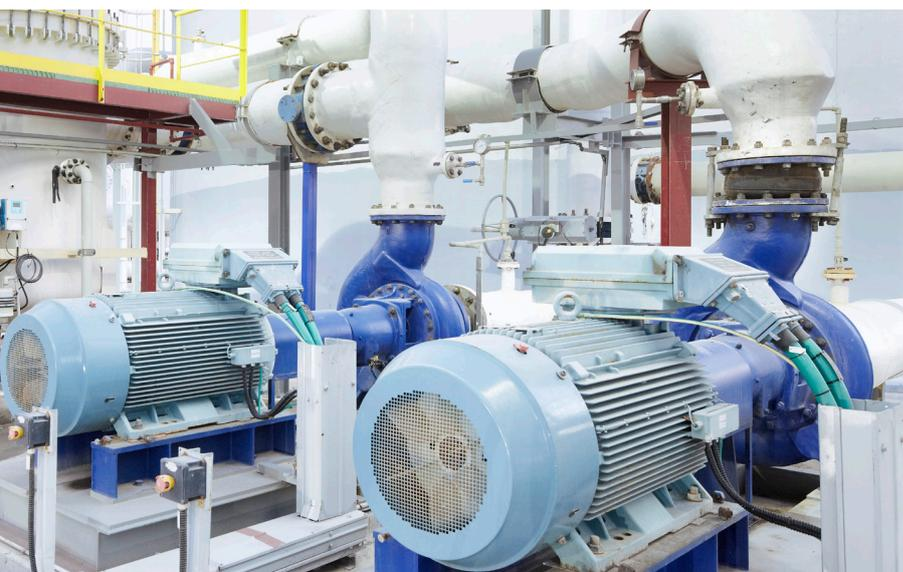
Thanks to ABB's softstarters having torque control, the issue of water hammering when stopping pumps was eliminated. Guhe Electric now saves \$30,000 annually.
