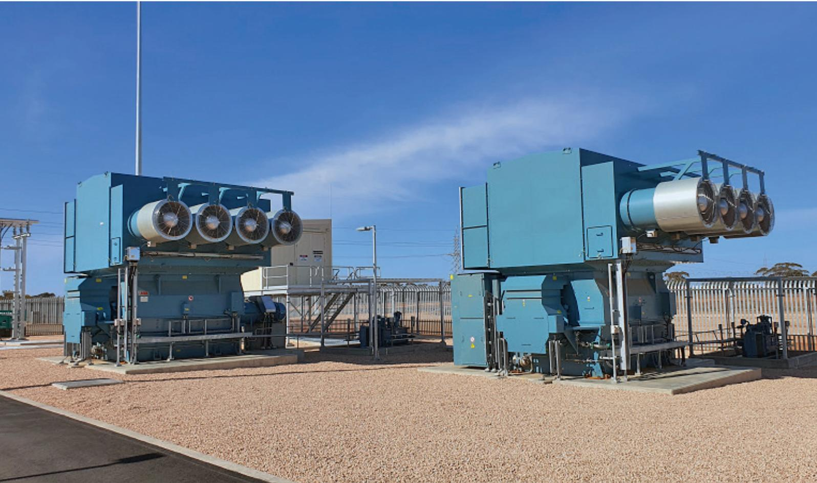
03 Darlington Point Solar Farm is supported by two ABB synchronous condensers at the farm's 132 kV connection point (image supplied by Edify Energy and Octopus Investments).
