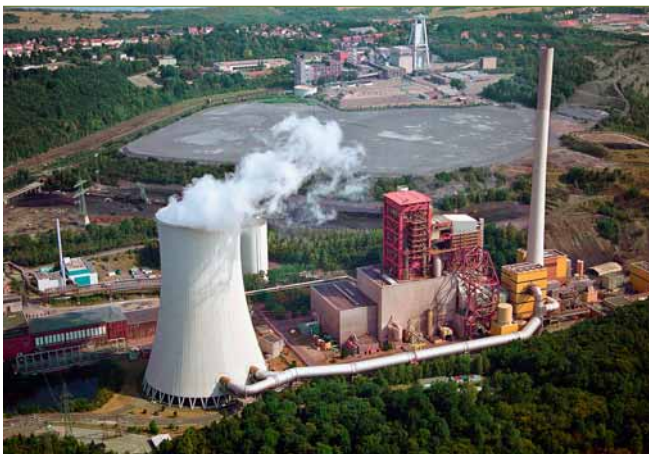
2 The Weiher III power plant, location of the first boiler startup installation
