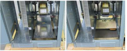
Then move the remaining sliding rail also below the power unit, so that it can be easily removed.
