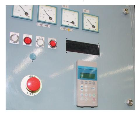
The picture shows an example of CDP 312 mounted directly onto an old Tyrak cabinet door.
