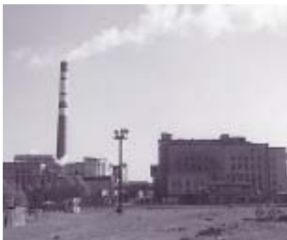
View of Horizon's pulp and paper plant in Kehra, Estonia.
