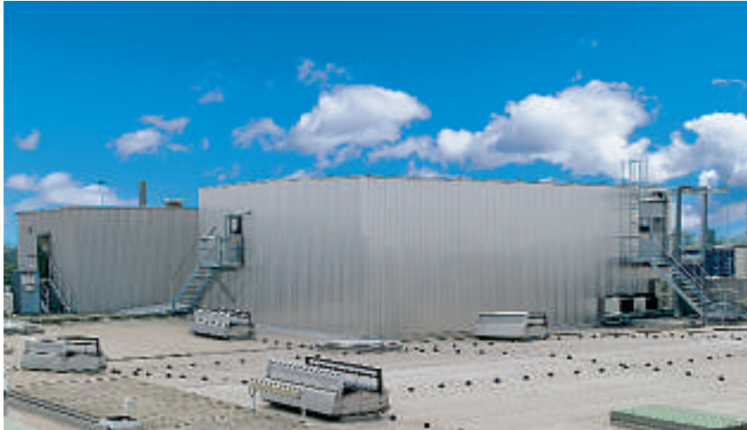
The new switchgear on the roof of the Opel factory
