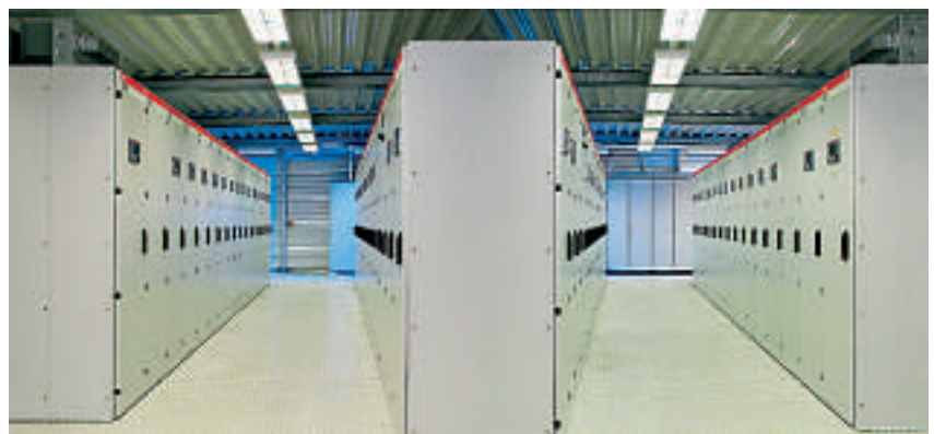
The 66 gas-insulated 20-kV cubicles of type ZX 1.2
