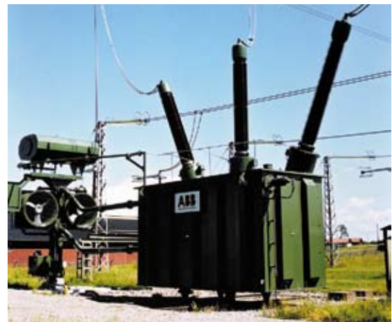
150 Mvar, 400 kV, 3-phase Shunt Reactor for the Swedish power transmission network.
