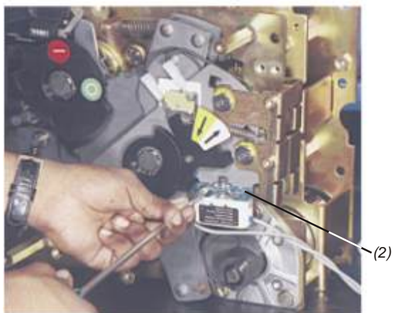
Steps For Replacement of Motor 15032
