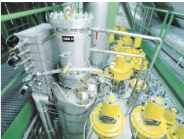
Lower cold box – the helium is cooled from 20 to 4.2 K and liquefied. Valves control the turbine pressure. From here the liquid helium flows (under the effect of the pressure difference) to the resonator cavities.
