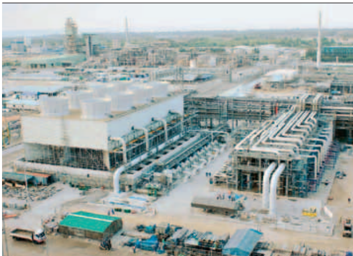
1 Thermoplastic polyolefin cooling area
