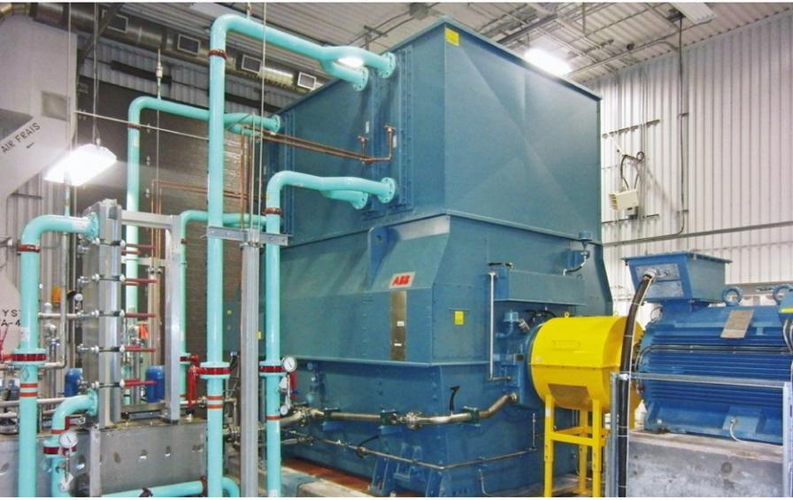
ABB is a global leader in power and automation technologies that enable utility and industry customers to improve their performance while lowering the environmental impact. Synchronous condensers from ABB ensure efficient and reliable operation of power grids through reactive power compensation and additional short circuit power capacity.
