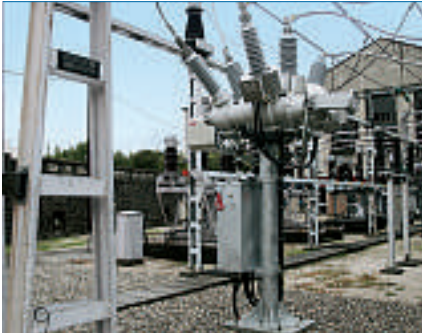
9 Active components on the structure.
