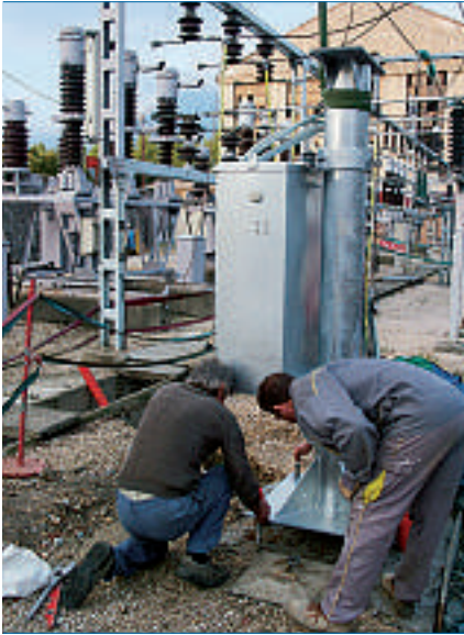
8 Installation of the supporting structure.
