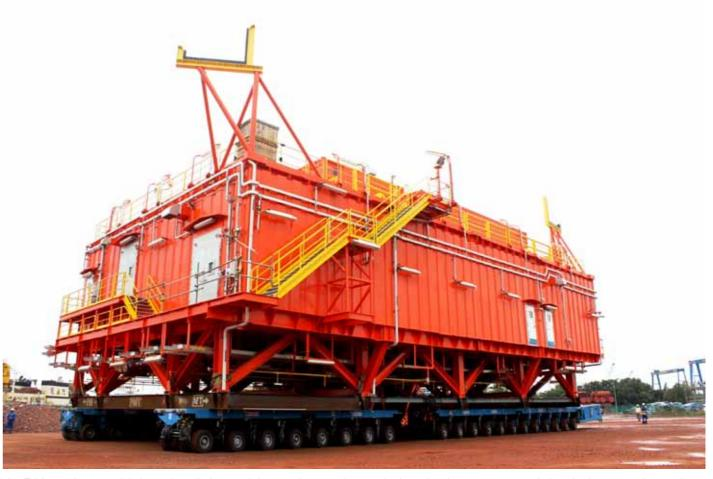
An E-House is a pre-fabricated, walk-in, modular, outdoor enclosure designed to house a range of electrical, automation and telecom equipment and ancillaries.
