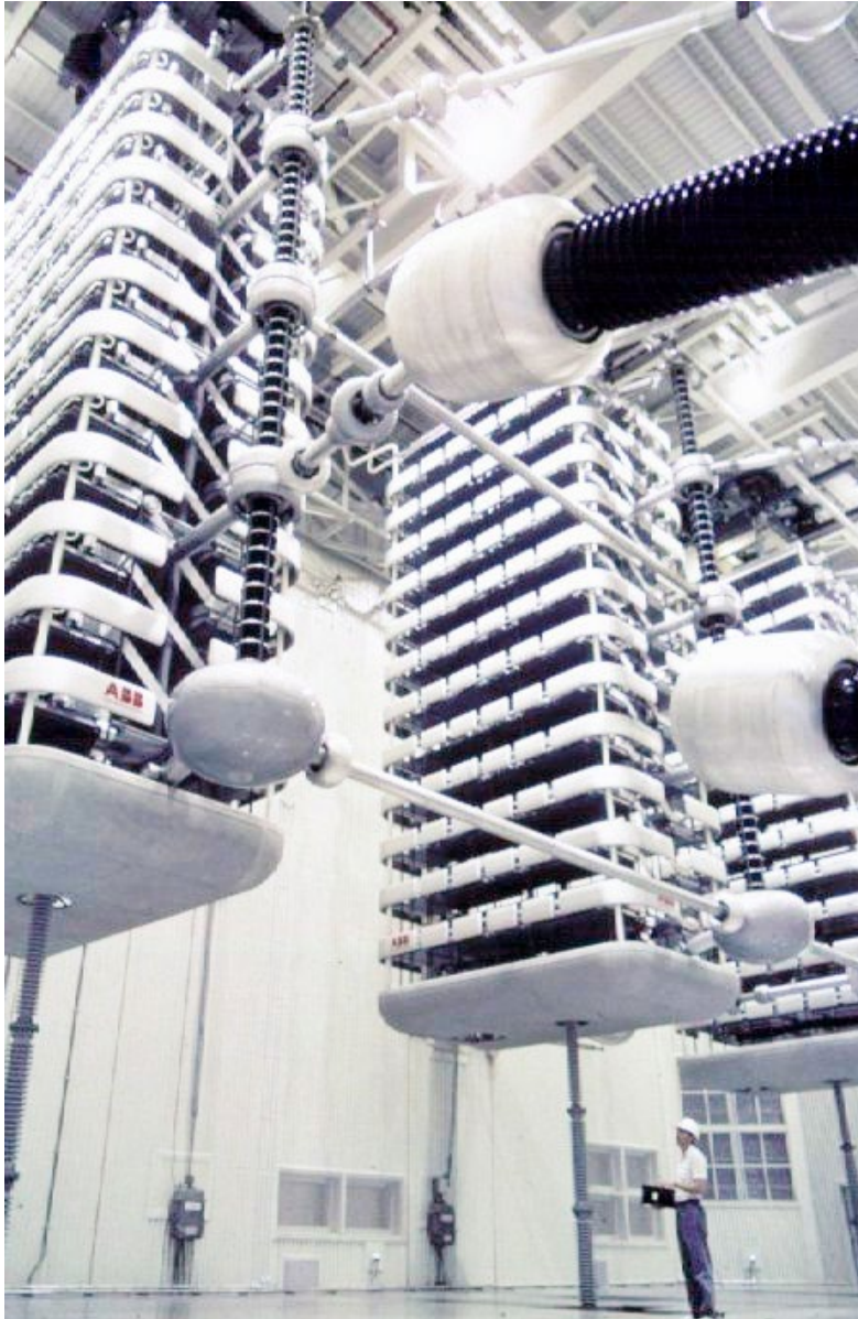
Figure 38: HVDC conversion station
