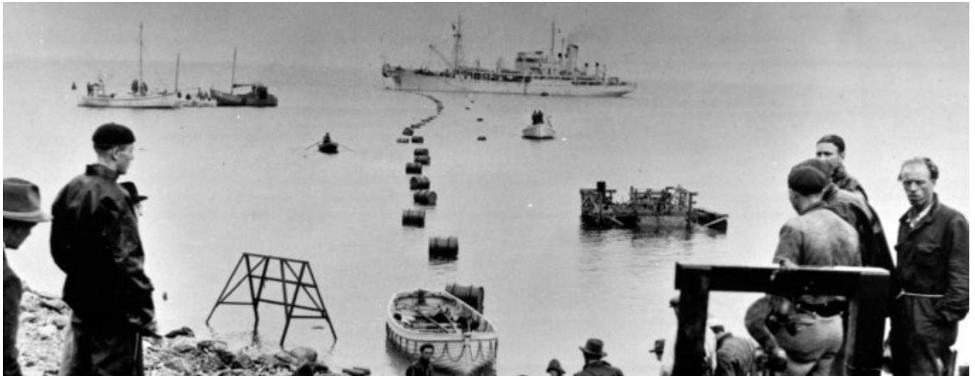
Figure 43: laying of an HVVDC connection in Gotland
