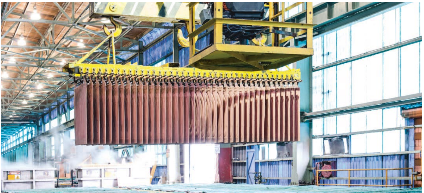
Figure 32: copper refining installation
