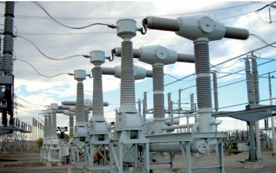
Hitachi ABB Power Grids high voltage service was hired to perform radiographic inspections of eight breakers for a Pacific Northwest utility in Fall of 2006. Using radiography to perform non-invasive diagnostic testing over traditional inspection techniques, reduced overall maintenance cost.
