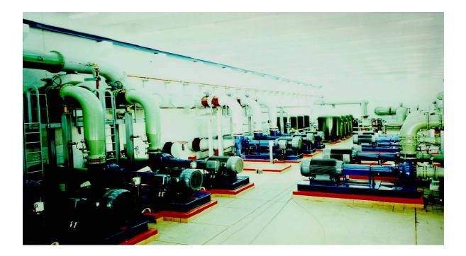
The New Dubai Sewage Treatment Plant is located 25 km from city of Dubai. Four sewage pumping stations 56,000-69,000 m<sup>3</sup>/d each are distributed over the city of Dubai and pump the sewage to a common pumping station of 260,000 m<sup>3</sup>/d where it is pumped to the treatment plant.
