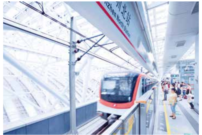
ABB also provides life-cycle service support including maintenance and retrofits for its large, global installed base.
