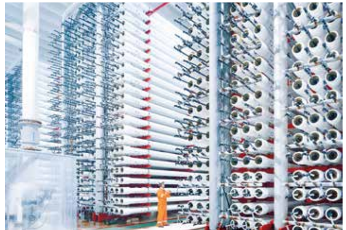
ABB drives are used in industries of all kinds, from cement to water purification (pictured) and help to boost process productivity, improve energy efficiency and cut maintenance costs.
