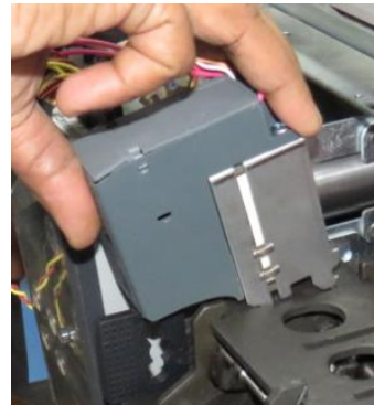
Figure 3. Shunt Trip inserting.
