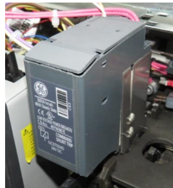
Figure 4. Shunt Trip assembly
