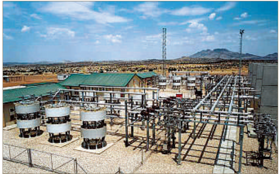
1 Auas static var compensator
