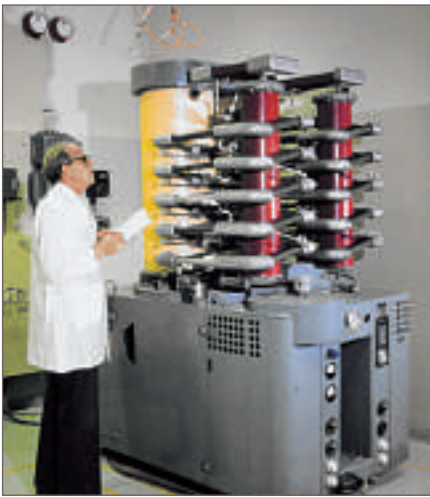
Early mercury-arc valve for HVDC transmission
