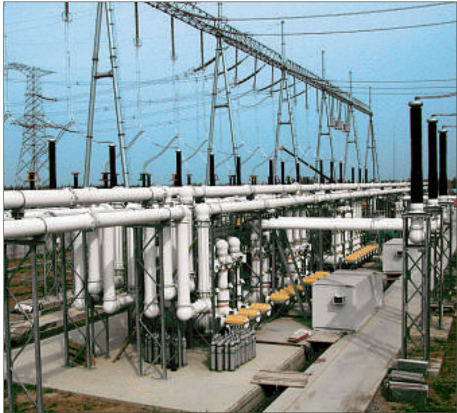
4 500-kV yard with SF 6 gas-insulated switchgear, at Jingzhou converter station (3GG)
