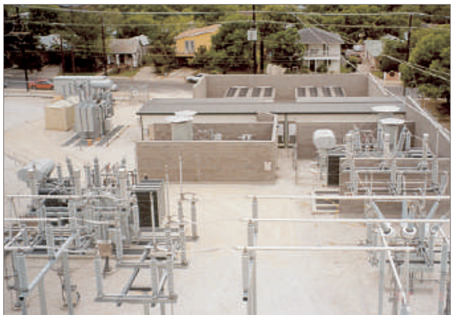
3 Eagle Pass back-to-back tie Foreground: 138-kV equipment and harmonic filters. Middle: buildings with converters, controls and auxiliaries. Back: cooling towers for water-cooled IGBT converters
