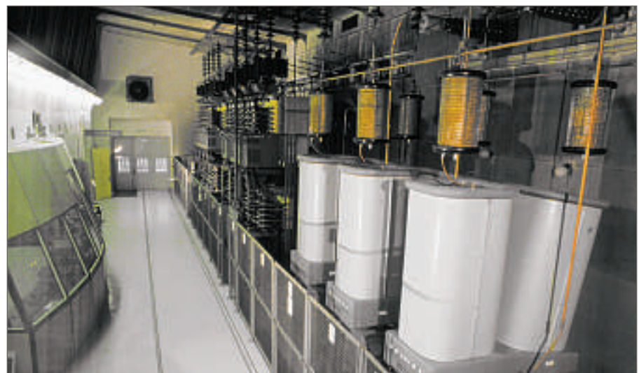
Gotland 1 extension, with the world's first HVDC thyristor valves
