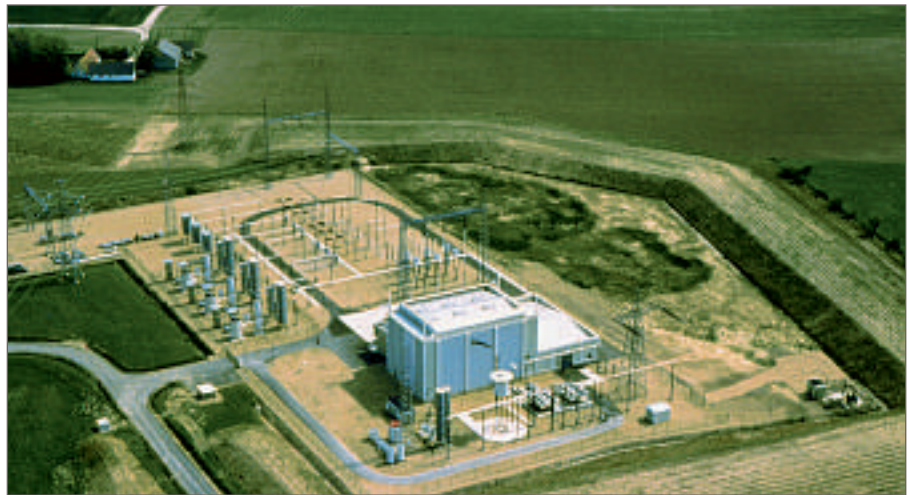
Baltic Cable HVDC converter station
