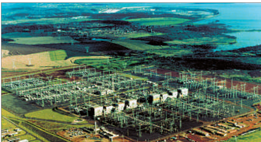
Foz do Iguaçu converter station with the Itaipu 12,600-MW power station in the background
