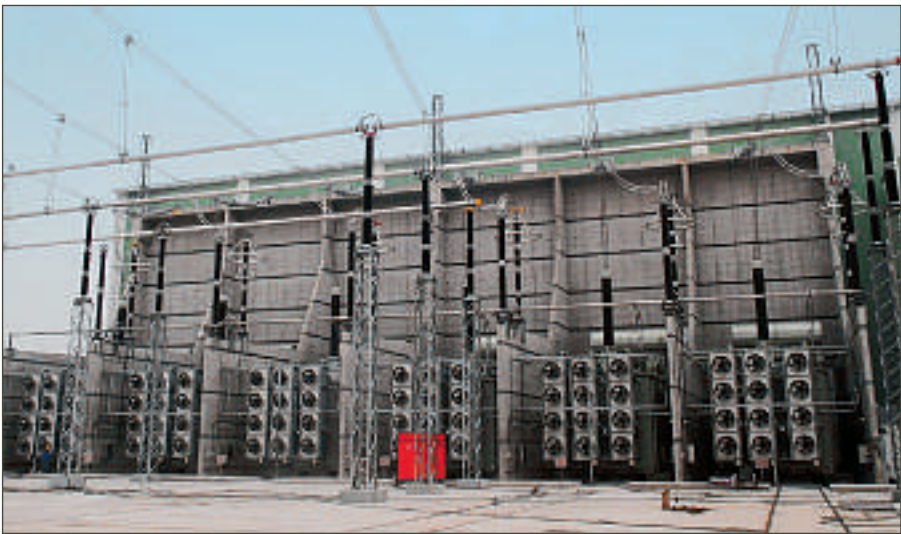
7 Converter transformer arrangement per pole
