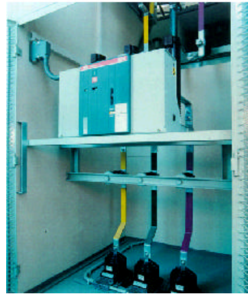
VD4 as a stationary-mounted unit in place of an air-blast circuit-breaker.
