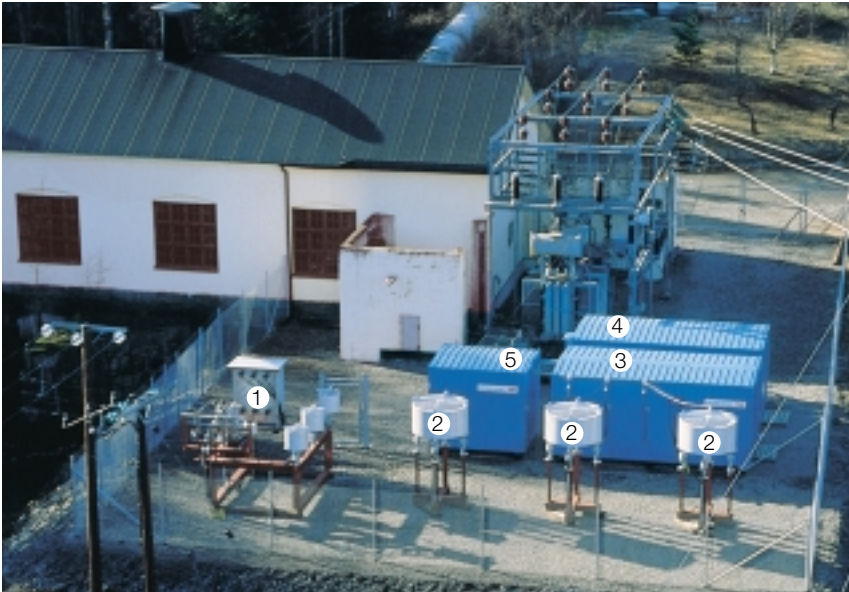
Hellsjön test installation in Sweden. The world's first HVDC Light transmission link is rated at 3 MW ±10 kV and uses a 10 km-long, temporarily decommissioned AC line. ❸
