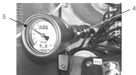
Fig. 2.3.1.1.3: Filling connector with pressure gauge (5) and locking ring (4)
