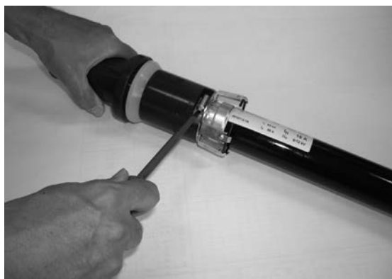
Fig. 4.3.5.7: Tightening the clamping band
