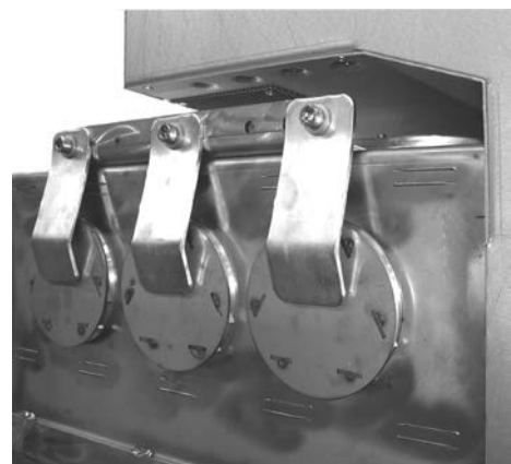
Fig. 2.3.3.1b: High dielectric strength blanking plugs in the busbar sockets
