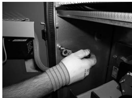
Fig. 2.3.2.9: Screwing the low voltage compartments together
