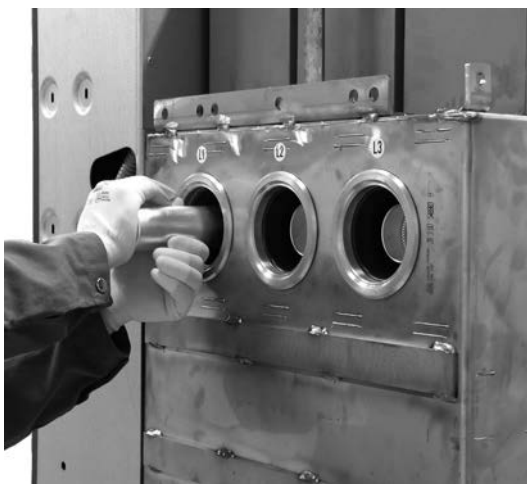
Fig. 2.3.2.3: Inserting a contact tube
