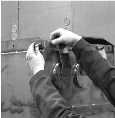
Fig.. 2.3.4.1: Fastening bracket for the end cover
