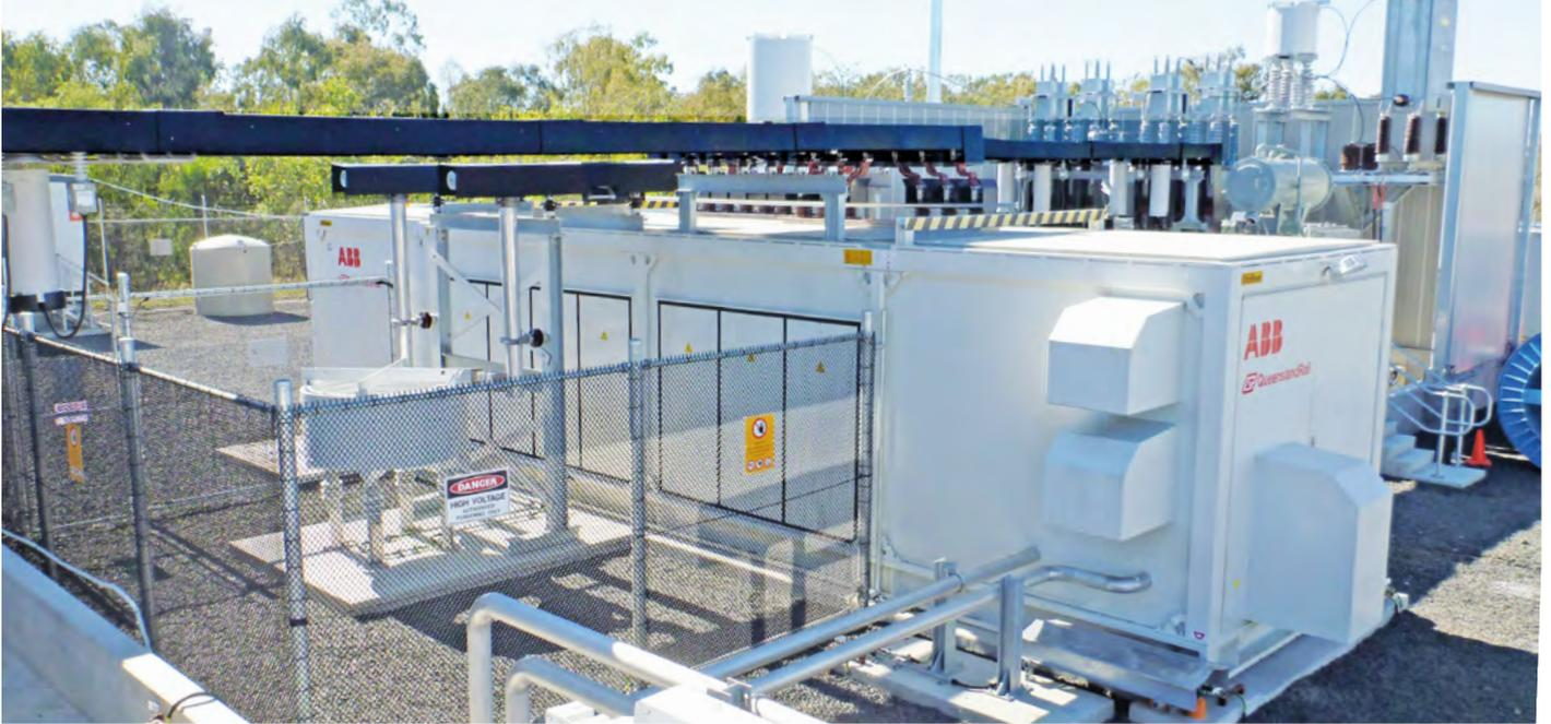
ABB is upgrading the feeder station at Wulkuraka in Australia as part of a program to strengthen the rail power supply for Queensland Rail's Brisbane suburban operations.
