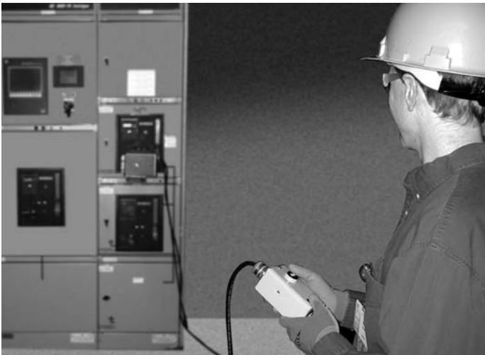
Figure 4.1 Remote Racking Operation
